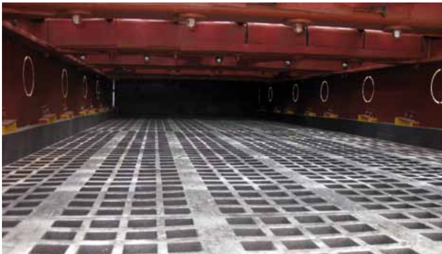
FS fitted with Trelex LS300 modular panels.
